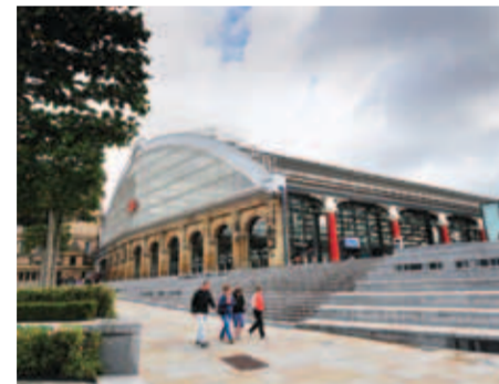
Liverpool Lime Street Station
